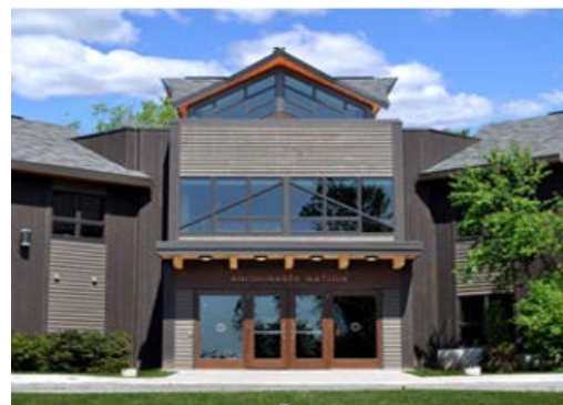
Union of Ontario Indians Administration Building
