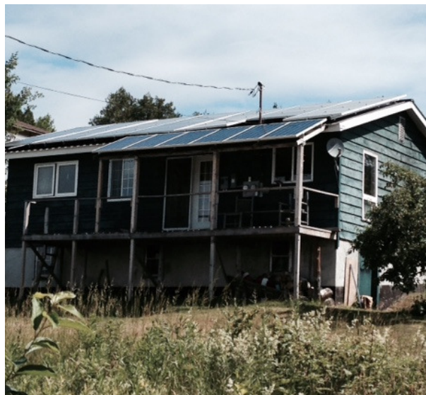
Figure 7. Bear Island Residence with 7 kw Solar Installation
